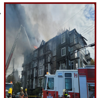
Structure Fire, Corbould Street April 2025
