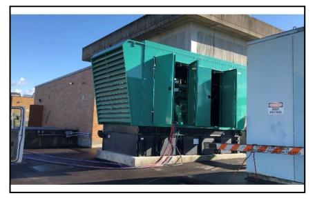
This fall, Operations installed a 750kilowatt standby power generator and new switchgear at the Wastewater Treatment Plant. Due to the growth and expansion of the plant it was necessary to increase the capacity of the existing generator to allow for treatment of sewage and general plant operations during power outages. Sizing and placement of the generator took into consideration existing site conditions, future expansions and long-term planning of the plant's electrical requirements.
