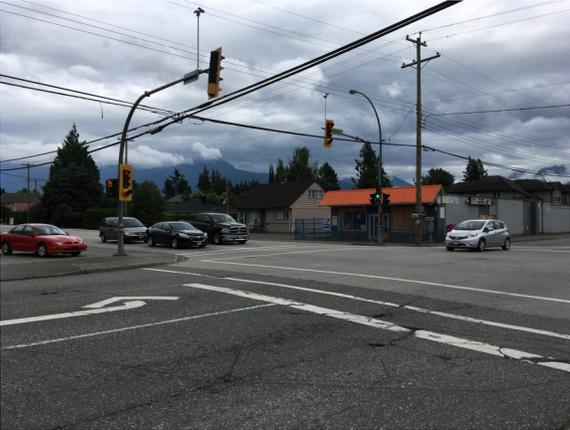
Pavement deterioration on all approaches led to traffic detection loop wire failures so a new video detection system has been installed. Video detection provides for continuous service even when asphalt is removed or damaged, it eliminates the need for loop wire cuts in the asphalt which accelerate deterioration and it is capable of detecting bicycles and small vehicles that loops typically miss.
