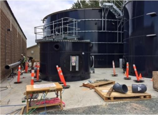
The project includes the construction of a high-strength wastewater pre-treatment facility (HSWWTF) at the City's Wastewater Treatment Plant (WWTP) to accept and manage high strength wastewater.
