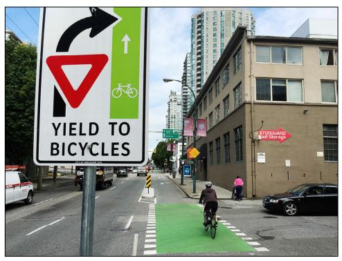
Figure 5.20 – Green pavement marking through intersection (Seattle WA)
