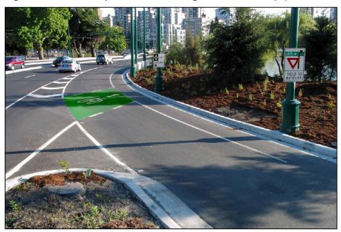
Figure 5.18 – Green pavement colouring in multi-use crossing (Canmore AB)
