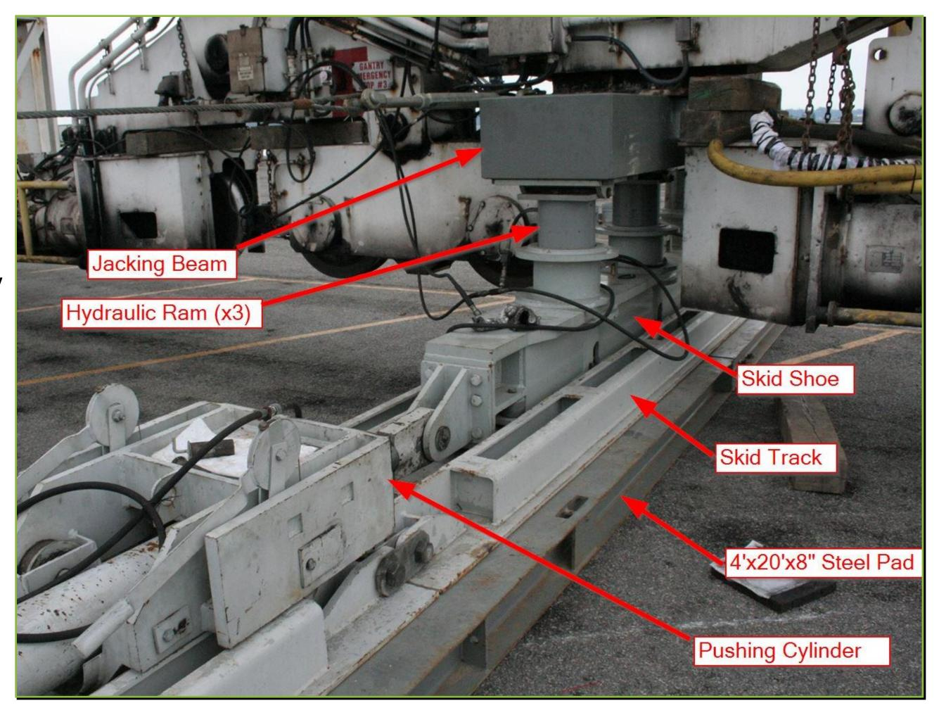
Although the bridge is 80 meters in length, the critical part of the launch is the first 60 meters when the bridge is cantilevered over the river, until the south end of the bridge touches down on the pier. It is anticipated that the first 60 meters of travel will be completed in one day. The remaining 20 meters of travel requires a series of detailed and coordinated steps and is anticipated to take two to three days to complete.
