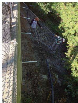
Shotcrete was placed along the footing portion of the lock block wall on Uplands Road (East) to prevent the loss of base gravel that had been migrating down the steep slope.
