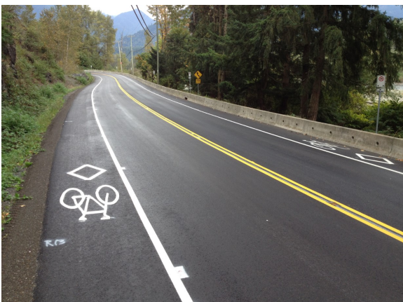
Chilliwack Lake Road - Overlay and Shoulder Paving
