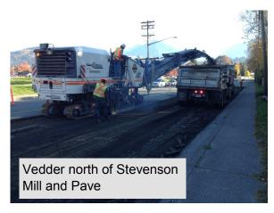
Keywest Asphalt Ltd has now completed the Asphalt Rehabilitation and Shoulder Paving program. A total of 10,738 tonnes of asphalt was placed on 16 roads with a cumulative length of 11.2 km.
