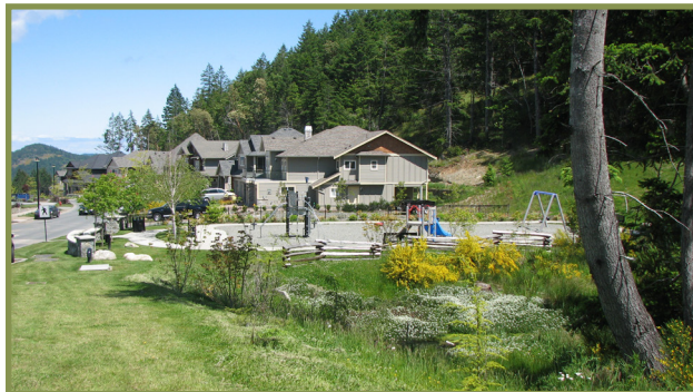
This wetland provides a valuable stormwater management function while also providing amenity space for surrounding residents.
