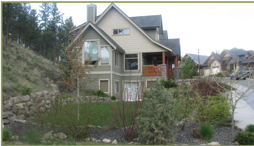
This lot configuration facilitates building orientation that runs parallel with the site contours. Combined with a reduced front yard setback, this configuration minimized grading requirements and preserved the site's hillside character while still providing usable outdoor space.
