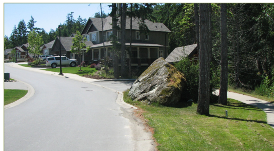
By adjusting road and sidewalk alignments, trees and a rock outcrop were preserved, adding to the natural quality of the development.
