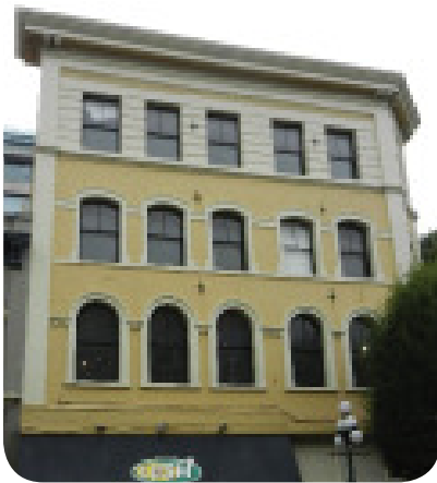
Photo 31 - Historic building with a distinct parapet treatment
