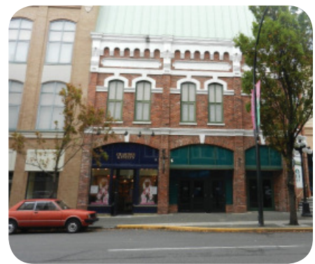
Photo 6 - Window size and façade treatments create contrast between the lower and upper levels of the building
