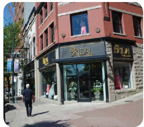
Photo 12 - Use of banding to emphasize building corner
