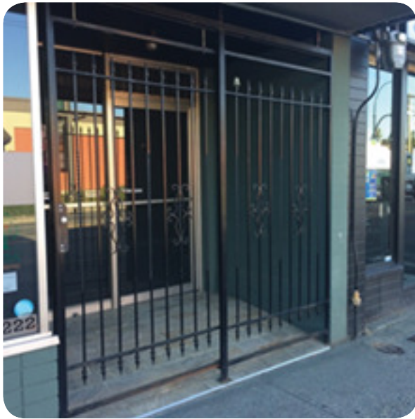
Fixed gate 100% transparent with ornate design showing detailing on bars and complementary colour to the building wall
