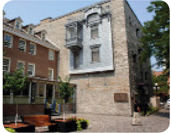
Photo 14 - Creative use of building forms to activate rear lane area
