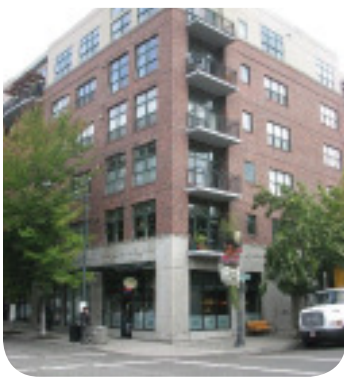
Photo 4 - Different materials and colours used to clearly differentiate between the lower and upper levels of the building
