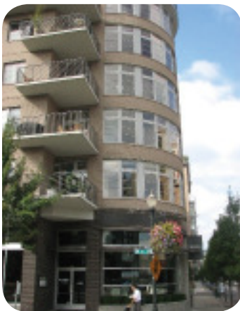
Photo 10 - Curved corner treatment
