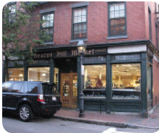
Photo 8 - Entrance that incorporates different treatment than rest of building
