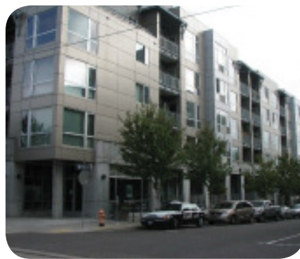
Photo 5 - Differing façade treatments between the upper and lower levels of development
