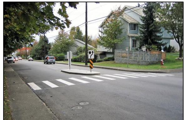
Figure M.4 Median Island at Crosswalk (North Vancouver)
