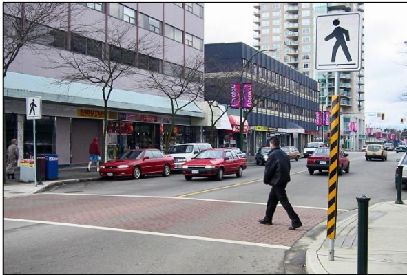
Figure M.3 Narrow Object Marker on Curb Extension (New Westminster)
