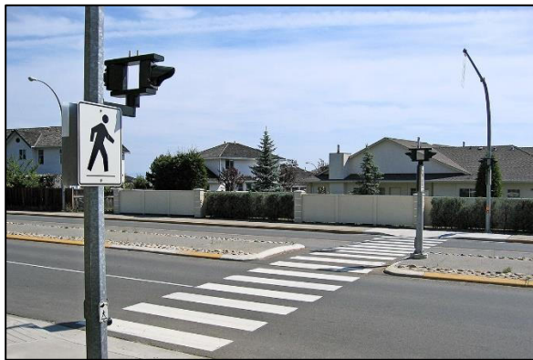
Figure M.5 Conventional Flashing Light Crossing (Nanaimo)
