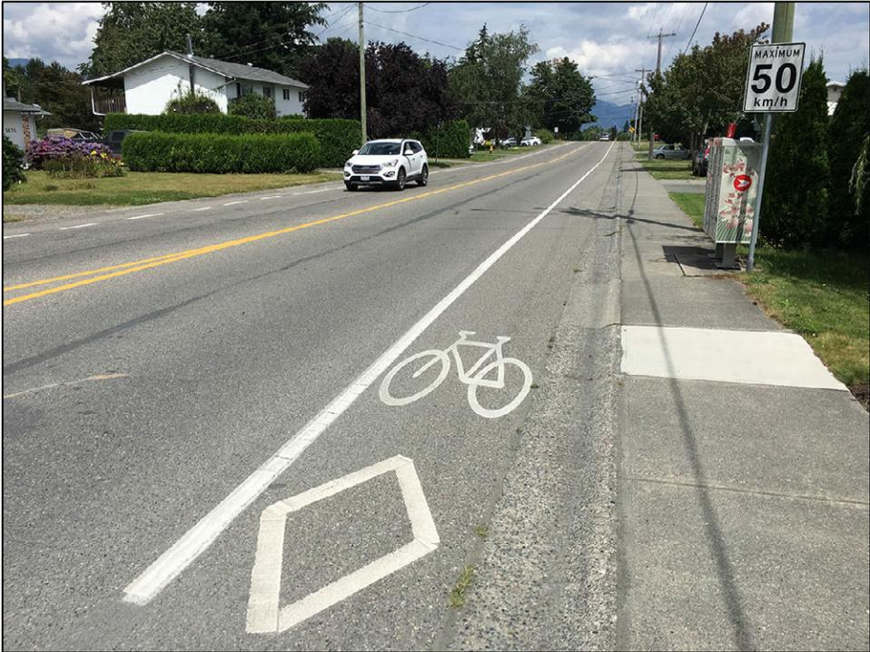
**Figure 2.3 – Buffered bicycle lane (Vancouver)**
