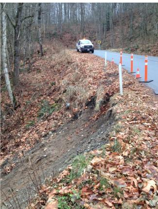
A slope failure at #46782 Thornton Road required a full road closure for a day and a half to armour the slope, place erosion control blankets and install a headwall at the culvert inlet.
