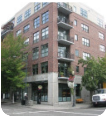
Photo 4 - Different materials and colours used to clearly differentiate between the lower and upper levels of the building
