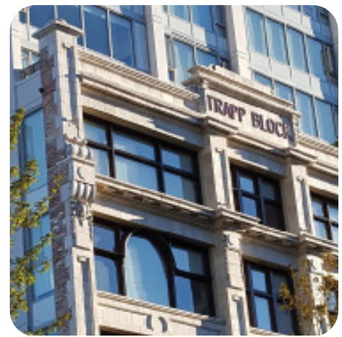
Photo 33 - Close-up of unique historic parapet treatment
