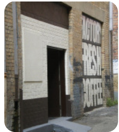
Photo 18 - Creative treatment of secondary façade
