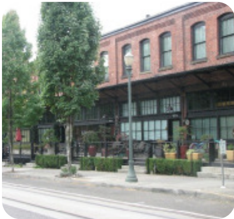
Photo 16 - Front façade treatment that contributes to the pedestrian environment
