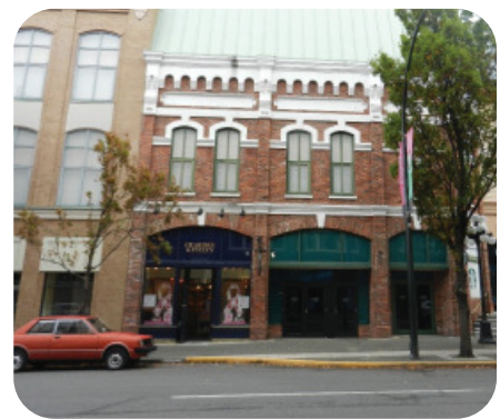
Photo 6 - Window size and façade treatments create contrast between the lower and upper levels of the building
