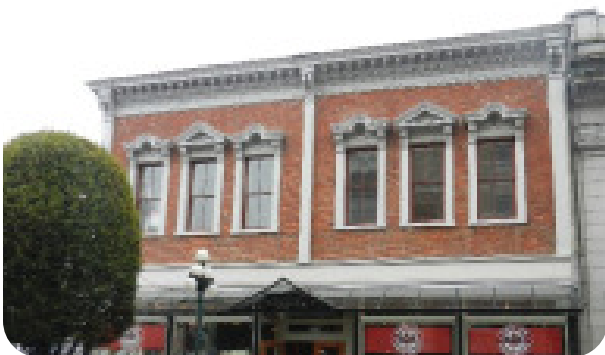
Photo 29 - Example of low-rise commercial building with flat roof
