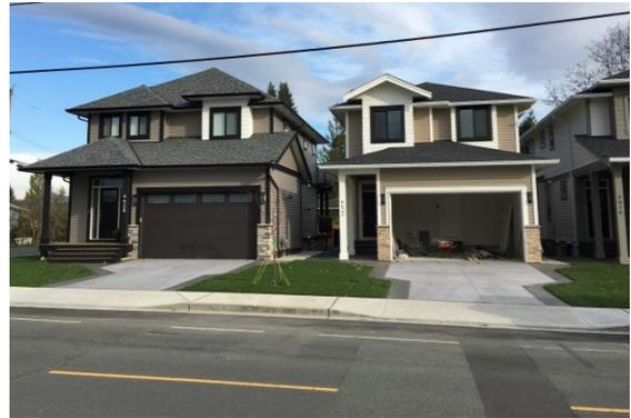
Example of driveways that are narrower at the road and widen to the width of the double garage once on the property. This protects the curb area for an on-street parking spot.
