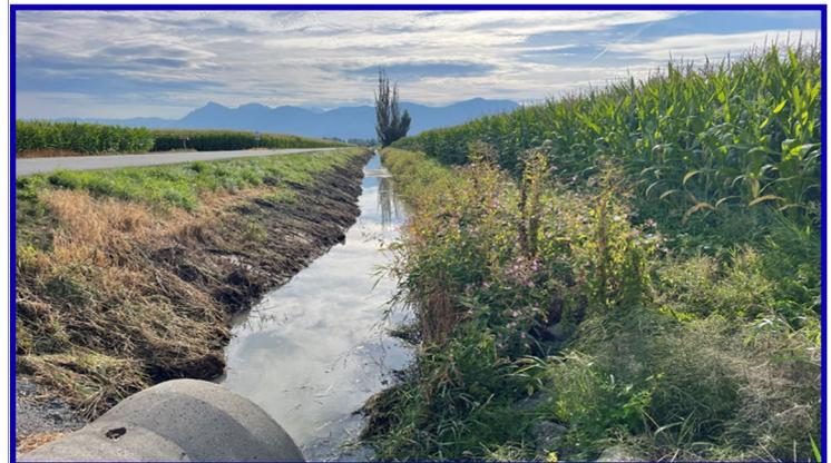
Atchelitz Creek channel conditions following channel excavation flood control work in August 2024. Note the removal of dense in-channel vegetation.
