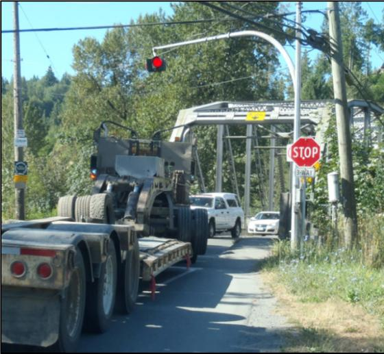
Width restrictions that are less than 100m in length may generally be referred to as “pinch points”. They should be eliminated on a priority basis as funds and other practical considerations allow. Signage and map notations warning cyclists of a pinch points allow them to plan alternate routes or be prepared to negotiate a potentially risky site.
