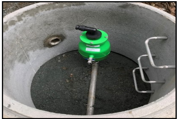
Patterson Road—New Sewer Air Valve
