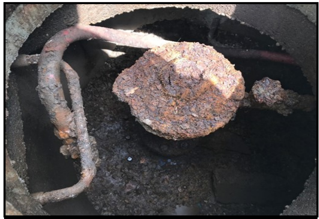
Patterson Road—Old Sewer Air Valve
