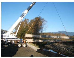
The pre-cast concrete girders are placed using a 500 ton capacity mobile crane. The Chilliwack Creek Division bridge is the shortest of two waterway bridges.
