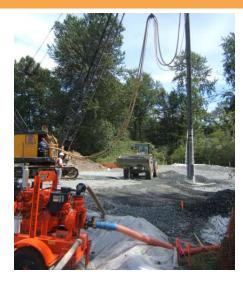
Bridge construction begins with foundation work. Underlying soils, as deep as 12 metres, have been strengthened with a soil densification process. This work will ensure post construction settlement is minimized.
